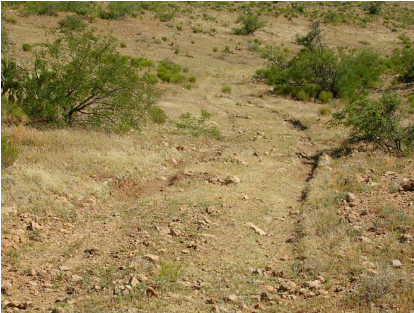
AC-10-06: Erosion on route Cw. Direction: S.
