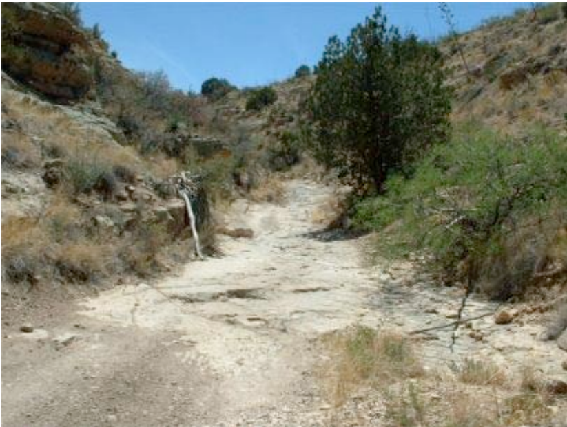
AC-B-07: Mechanical improvements on route B (Grinding of road bed and left hand cliff wall). Direction: SW.
