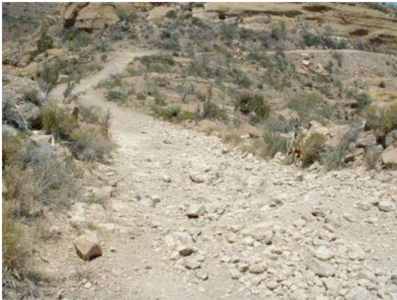
AW-B-05: Erosion on route B. Direction: S.
