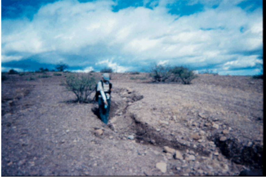
Th-20-17: Worst erosion on route Cu. Direction: NE.
