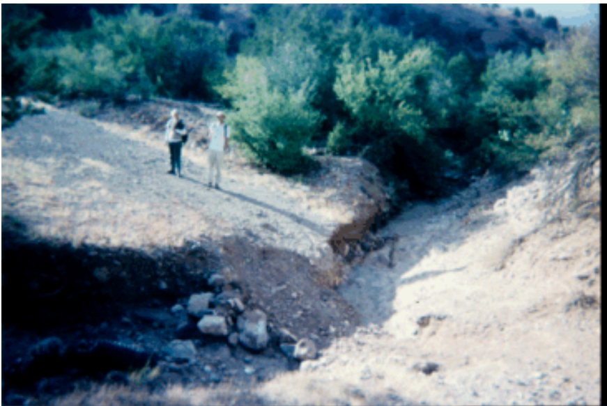
Th-20-07: Severe erosion where route Cx crosses a deep gully. Direction: SW.
