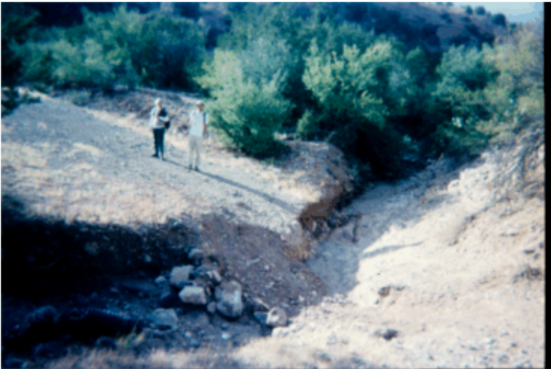
Th-20-07: Severe erosion where route Cx crosses a deep gully. Direction: SW. T 6S, R 19E, Sec. 5. UTM: 553157E, 3645215N, Datum NAD 27.
